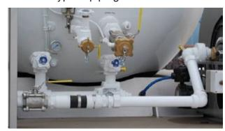
Meter discharge piping includes stainless steel ball valve (flanged body) with flexible connector and swivel adapter.
